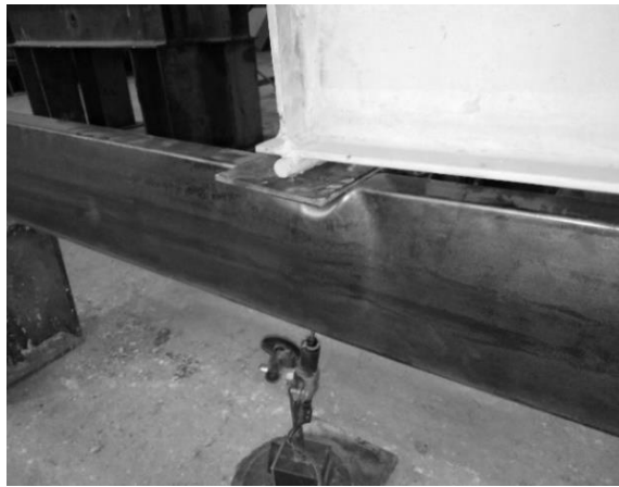
A.) EXPERIMENTAL FAILURE MODE.
