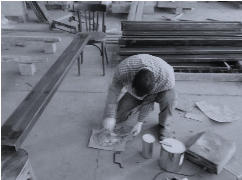
FIGURE 4. MIXING AND APPLYING OF ADHESIVE RESIN ON STEEL SURFACE.
